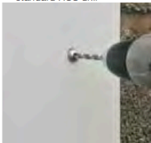
E. Drill out Hex socket using standard HSS drill
