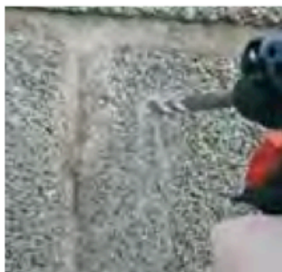
A. Pre-drill base material
