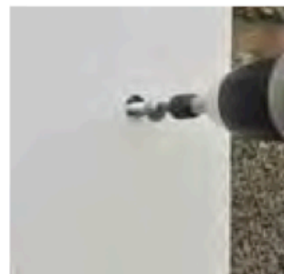
C. Position fixture, tighten bolt into shield
